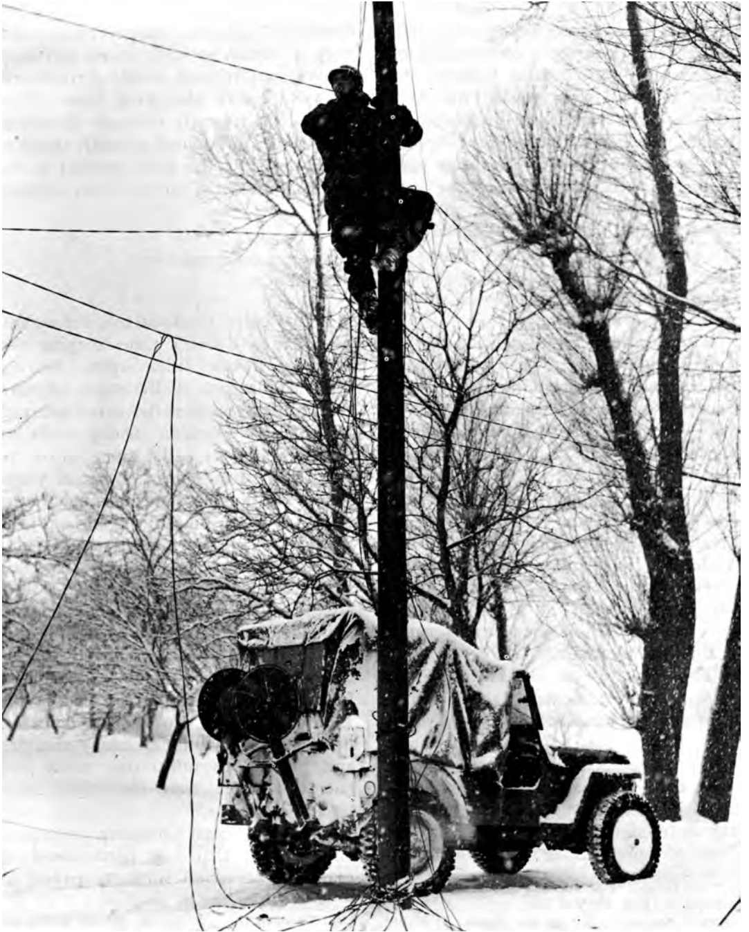
SIGNAL LINEMEN REPAIR WIRE IN THE ARDENNES
