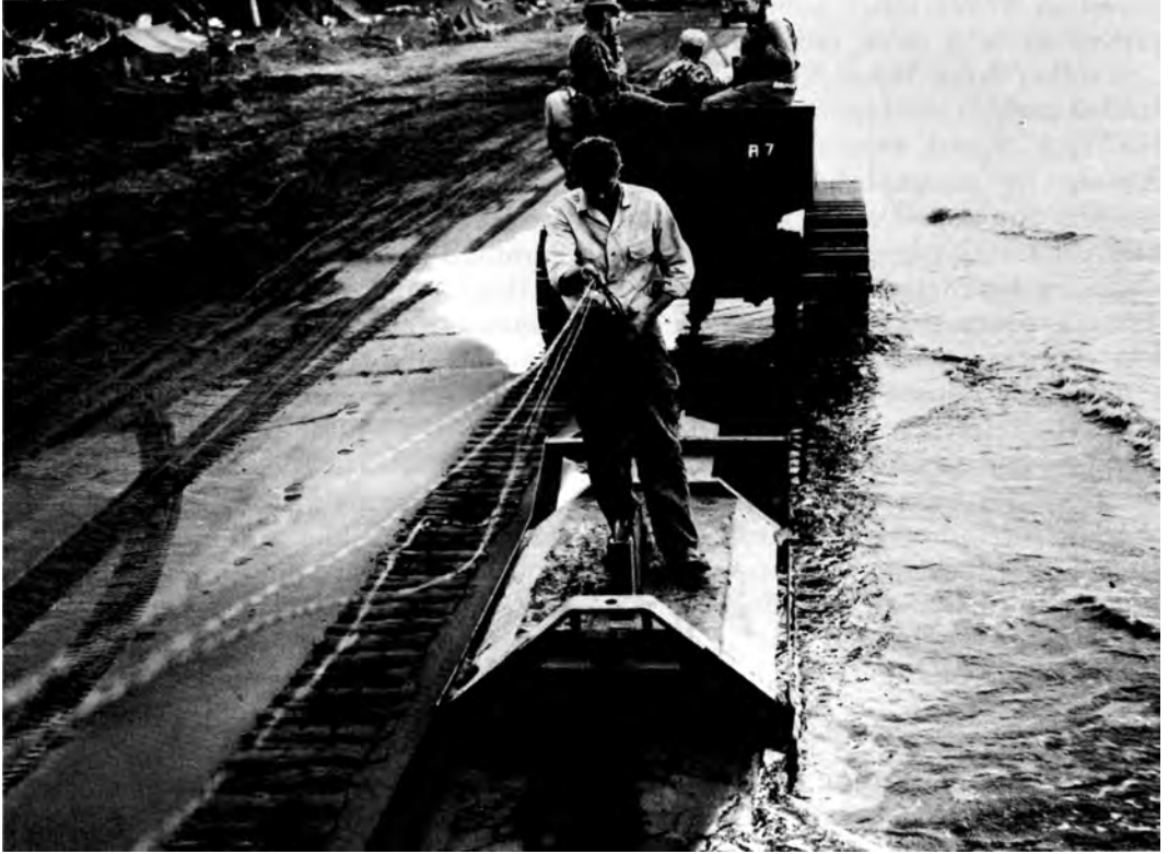
PLOWING IN CABLE AT THE WATER'S EDGE, HOLLANDIA
