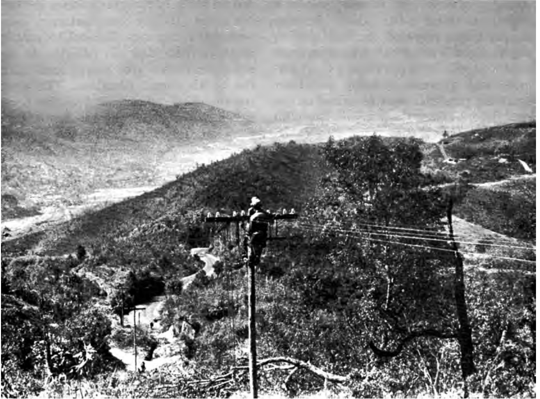
SIGNAL LINEMEN STRING WIRE BESIDE THE STILWELL ROAD
