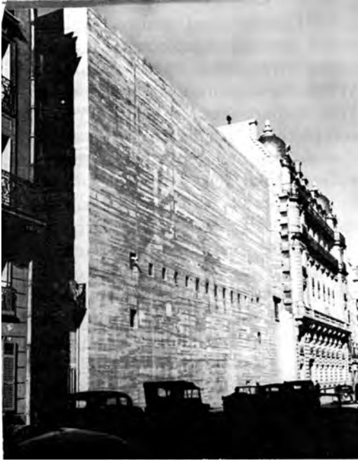
PARIS SIGNAL CENTER in German-built blockhouse.
