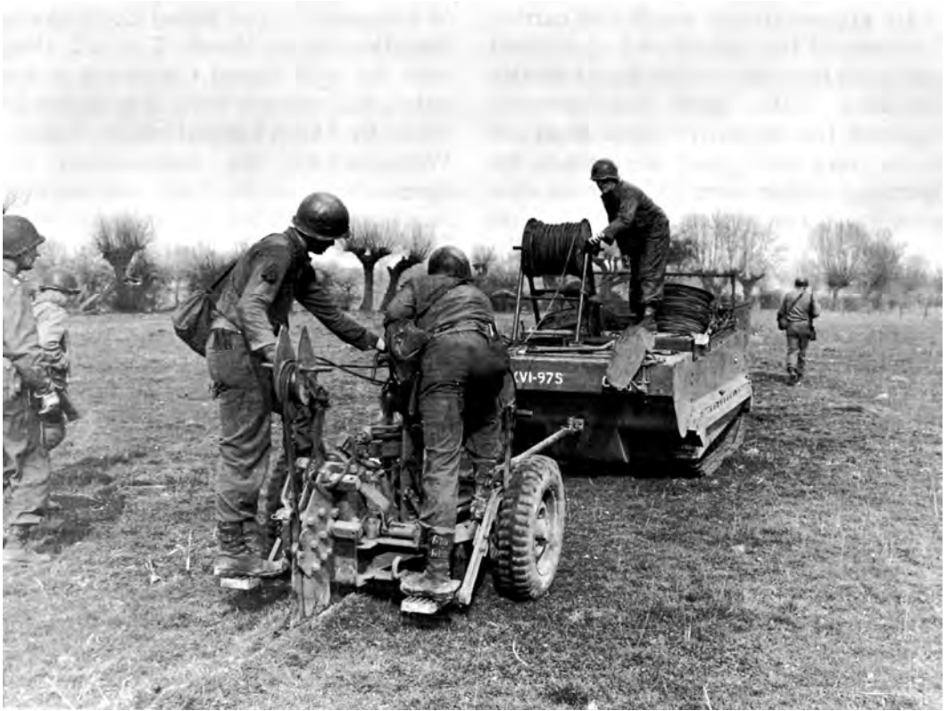
BURYING SPIRAL-FOUR NEAR THE RHINE WITH A CABLE PLOW
