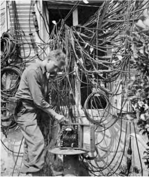
NEW DEVELOPMENTS IN SIGNAL COMMUNICATIONS included spiral-four cable (left and right above) and the BD-100 teletypewriter switchboard (below), with three TG-7 teletypewriters.
