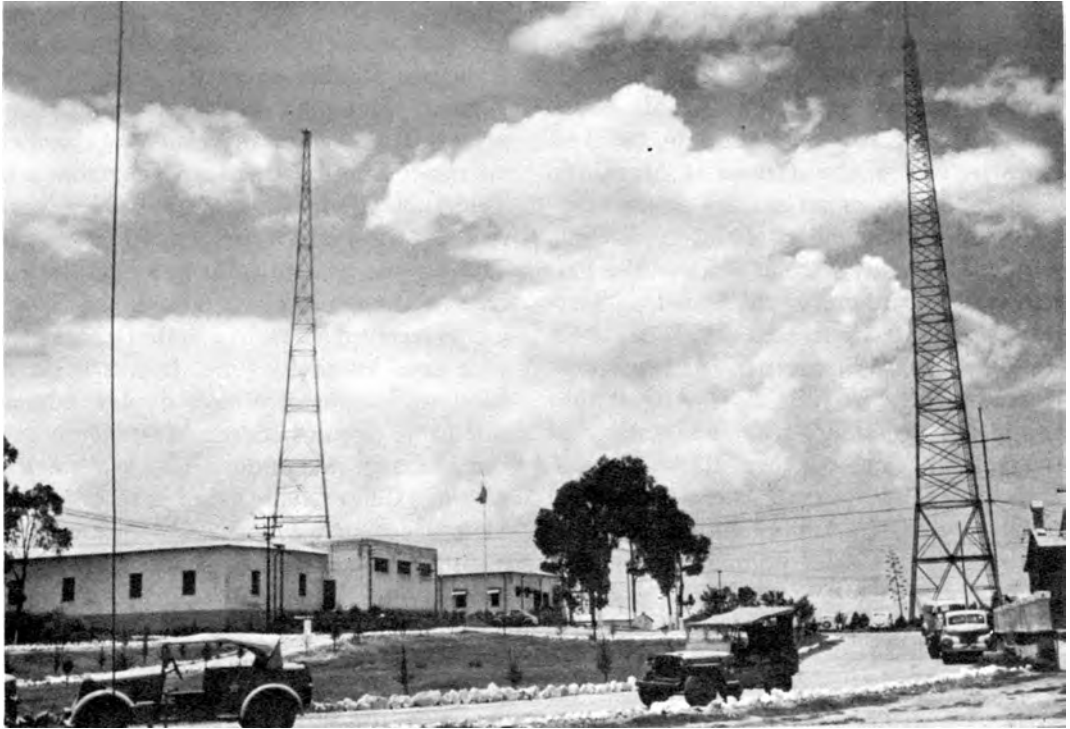
ANTENNA TOWERS OF RADIO MARINA, ASMARA
