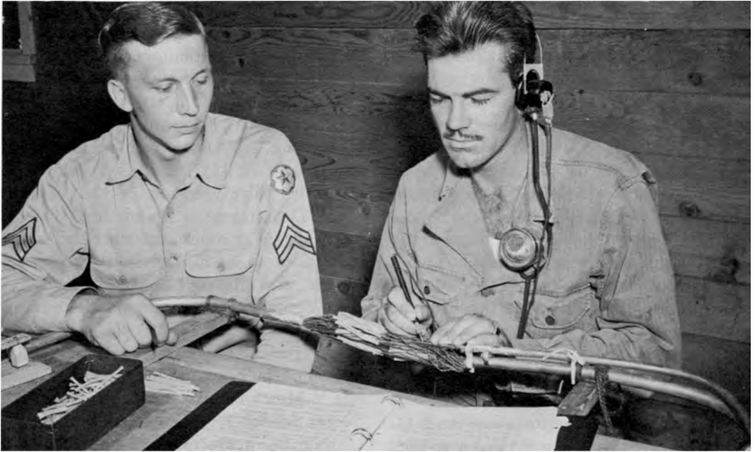
TRAINING AT CAMP CROWDER. Cable splicing (above) and message center operation (below).
