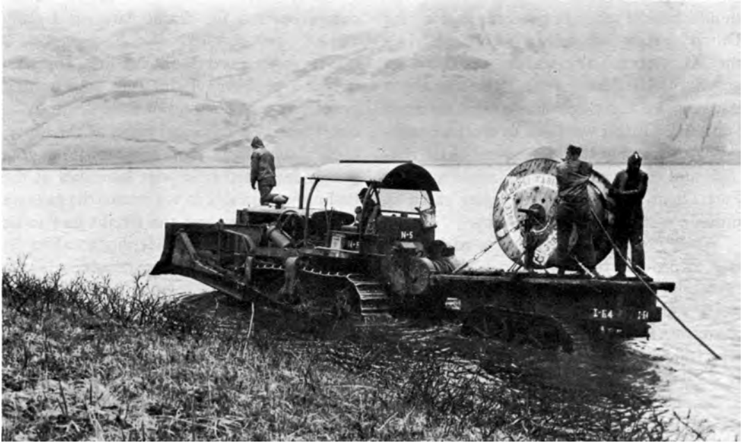
CABLE-LAYING OPERATIONS IN ALASKA. Cable is shown being laid along the shore at Fort Mears, above. Below, the cables ship Restorer.
