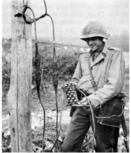
NEW DEVELOPMENTS IN SIGNAL COMMUNICATIONS included spiral-four cable (left and right above) and the BD-100 teletypewriter switchboard (below), with three TG-7 teletypewriters.
